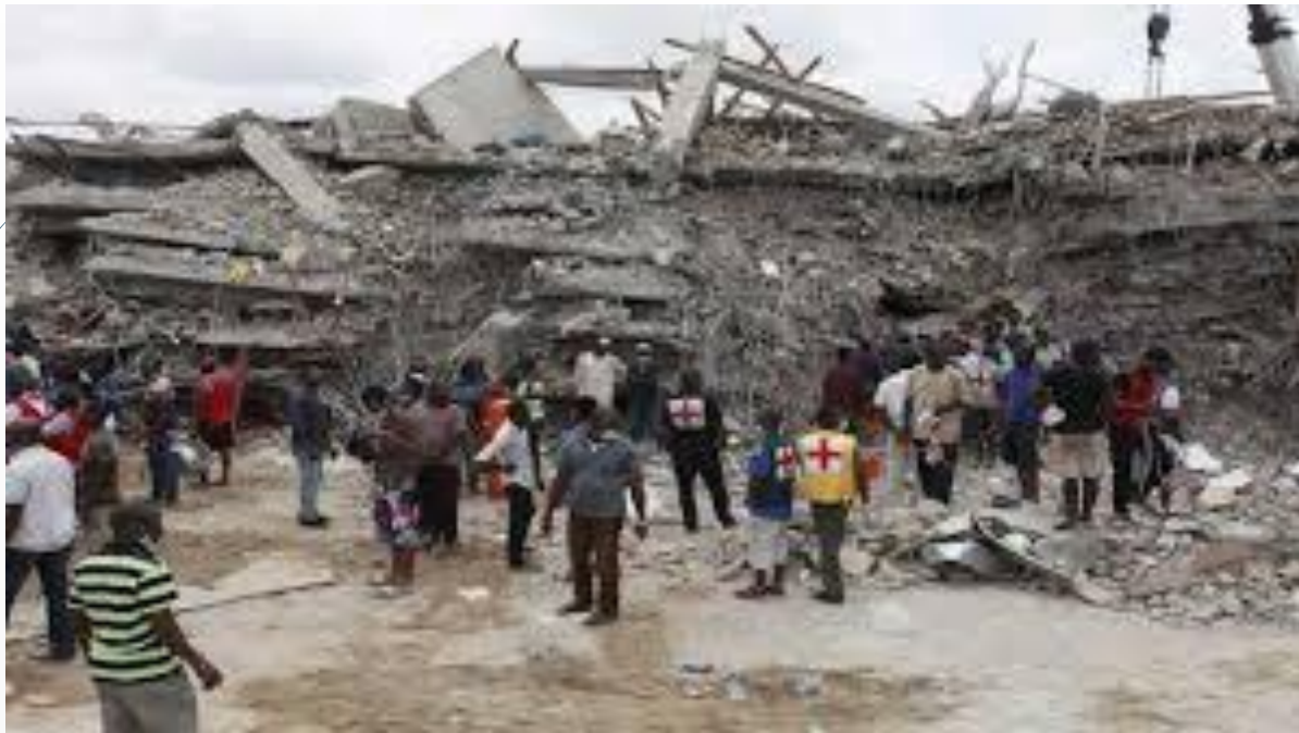
Plate II: 6 Storey Synaguoge Hostel Building Collapse that Claimed 116 lives
