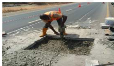
Destructive testing with Demolition Hammer, with shovel, diggers and hoes
