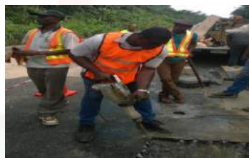
Destructive testing with Demolition Hammer, with shovel, diggers and hoes
